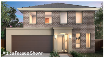
Attica Facade Shown
